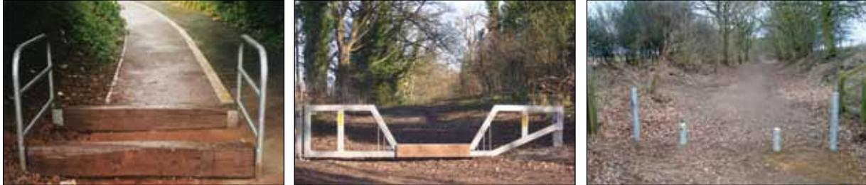
*Left, horse stile – prevents motor bike use - and, centre, horse-friendly vehicle barrier (photographs by kind permission of Centrewire); right: Kent Carriage Gap (photograph by kind permission of Maydencroft Rural Ltd. See appendix for contact details and Kent Carriage Gap specification).*
