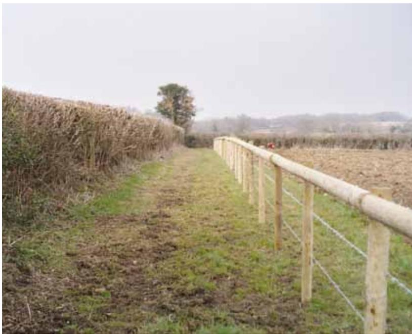
The fenced-off section leading to the green lane and exit in Whatley was provided to prevent users trespassing across the middle of the field. Posts erected with a single rail on the inside and wire on the outside for horse safety and to facilitate change of land use to keeping cattle in field at later date. The tenant allowed ample width to facilitate hedge cutting and mowing. This section is a new bridleway creation and benefits walkers by linking existing PROW.
