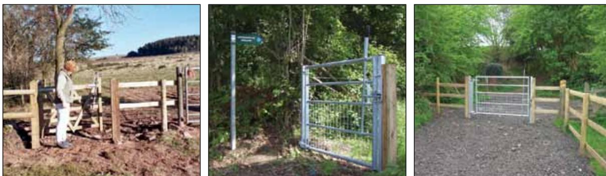
*Left, Fountain Timber wooden gate with Centrewire fittings; centre, Chiltern galvanised gate with one-way opening mechanism and stock-proof handle; right, Chiltern galvanised gate with two-way opening mechanism and straight easy latch handle. Chiltern photographs by kind permission of Centrewire (see appendix for contact details).*
