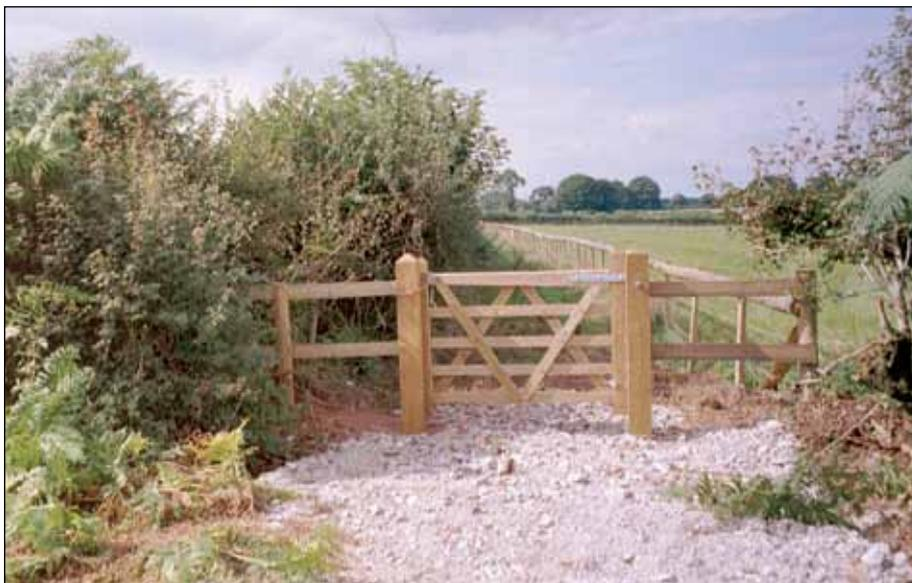
*Section of community trail at Binegar (see TTT case study 2, guide section 23). This new bridleway at Rookery Farm crosses land where horses and cattle are kept and is close to a busy main road. It has been fenced with posts and inner top rail and field side stock proof fencing to form a safe user corridor to separate users from stock and to ensure stock security.*
