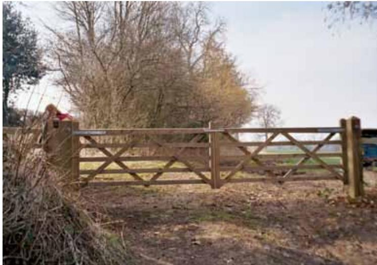
New bridleway entrance from the two track rural road has been constructed. There is ample room for users to enter or exit before or after crossing the road to or from the verge on the other side leading to the Fordbury Lane section of the trail. The barbed wire Wiltshire gate has been replaced with a pair of wooden estate gates plus a 5ft one-way bridleway gate closing against the boundary has replaced the original kissing gate.
