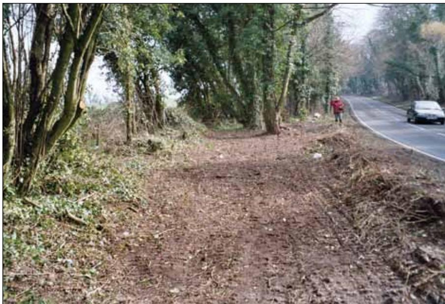
*Works were carried out to clear the verge to facilitate direct crossing instead of staggered crossing and to improve visibility. The Murder Combe proposed route survey defined it as priority 1 because of its importance to the network as a crucial link in both a community and linear trail.*
