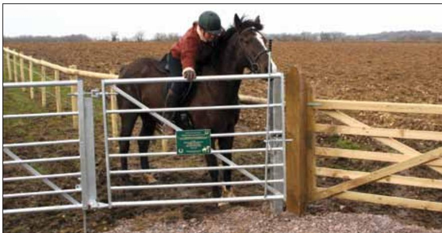
*Dual-purpose Centrewire York gate at Murder Combe with a two-way opening bridleway gate and integral vehicular gate section that can be locked to prevent unauthorised use. A new entrance into this field has been created (on right). The stock-proof fencing erected has barbed wire on the field side but the horse and rider are protected by the rail on the inside.*
